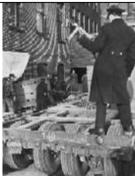
1958 Vault Installation Concord Savings Bank (Herbie Norton)
